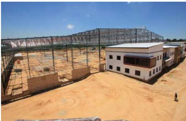
**Renico Construction’s speculative construction of a new 22 500 m<sup>2</sup> warehouse with offices in Mostyn Park X1 during 2011. The hybrid structure was manufactured and erected by Robor**
