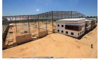
Renico Construction's speculative construction of a new 22 500 m<sup>2</sup> warehouse with offices in Mostyn Park X1 during 2011. The hybrid structure was manufactured and erected by Robor
