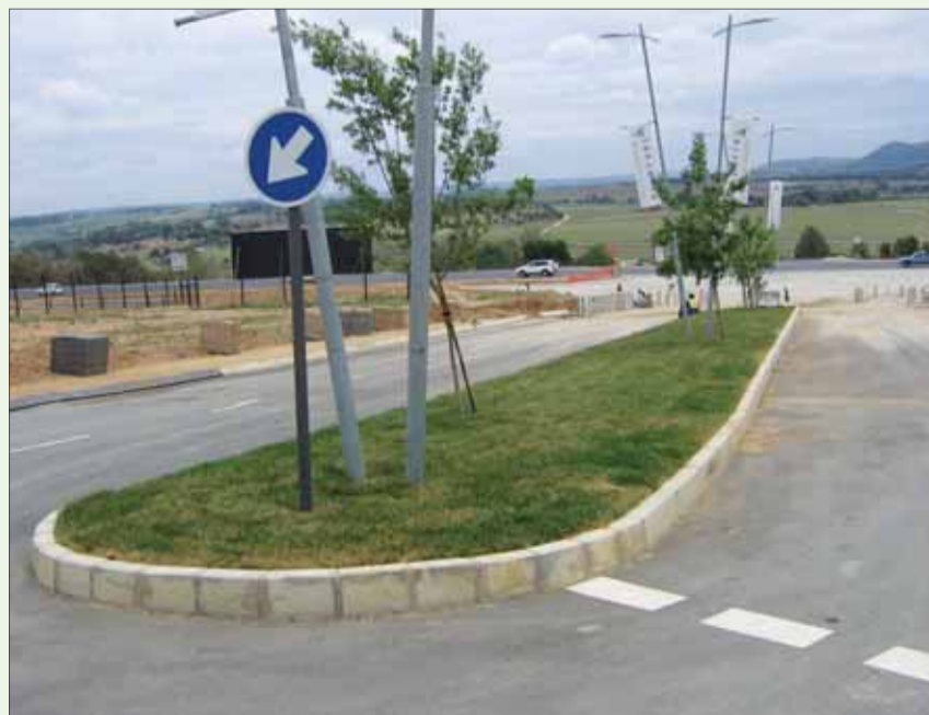
Road upgrades surrounding Lanseria Corporate Estate
