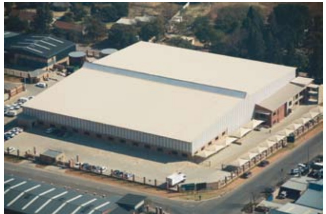
Aerial view of the UTI/Sun Couriers warehouse building
