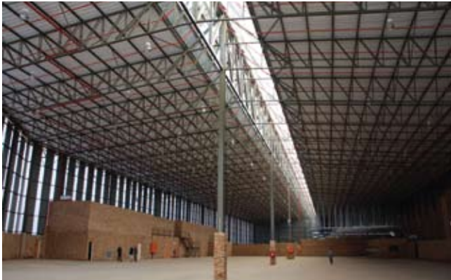
Pictured is the traditional structural steel used at the Lasercom building and the UTI/Sun Couriers warehouse building
