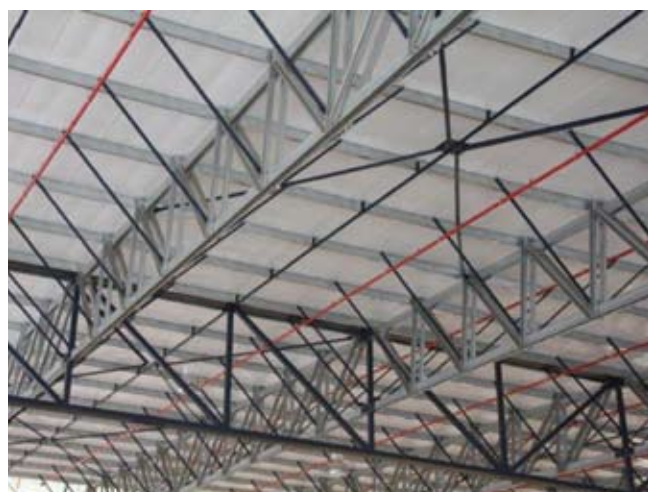
Interior view of the lightweight hybrid structure inside the Eureka DIY II 800 m 2 factory in Lea Glen X2, Roodepoort, Gauteng
